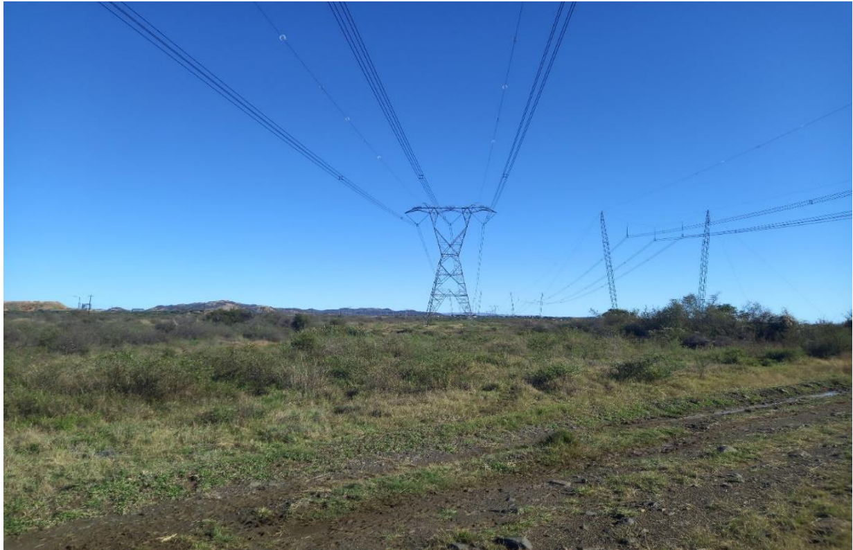
Figure 9: View of the powerlines noted on the margins of the site.
